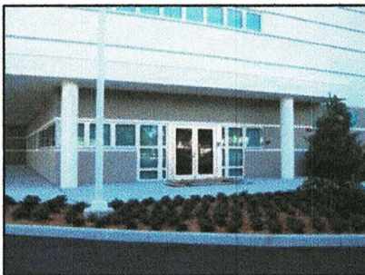
Figure 5. St. Charles Emergency Operations Building, LA
